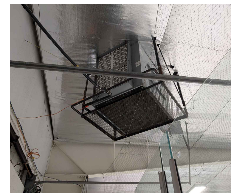
REFERENCE IMAGE - EXISTING DEHUMIDIFIER WEST ELEVATION
