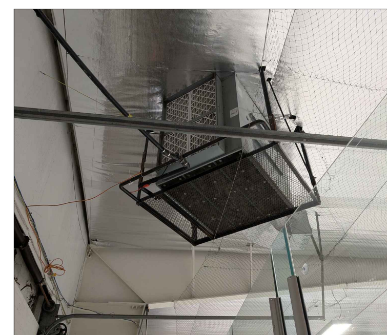
REFERENCE IMAGE - EXISTING DEHUMIDIFIER WEST ELEVATION
